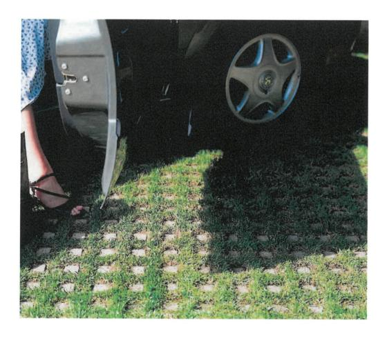
Images of C35. A plastic grid concrete is poured into and then when set the plastic is burned away. The burning bit is probably not great for the environment.
